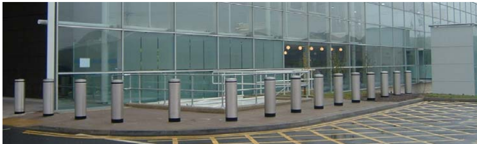
Installation completed with the addition of aesthetic sleeves.
